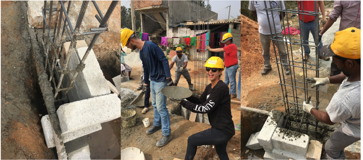
Figure 3: Pouring the footings at house #1 using the “bucket brigade”
