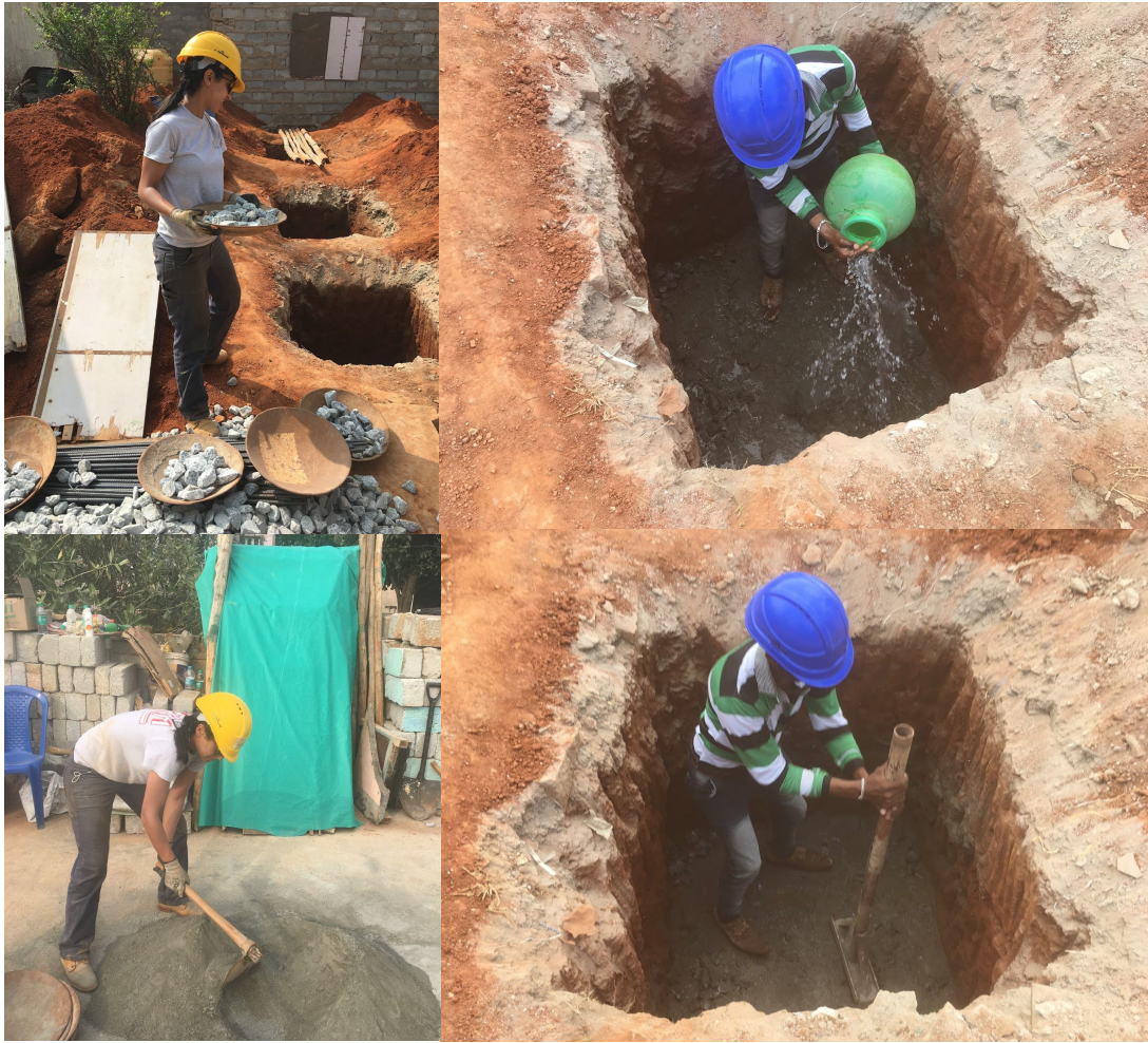
Figure 2: Pouring the footing at house #3
