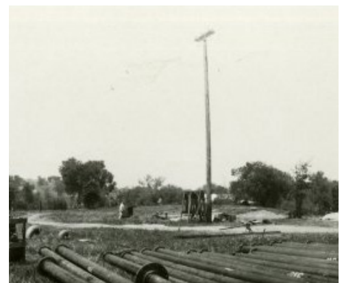
Steel pipes being prepared to construct water mains (Atascadero Historical Society, 1915).
