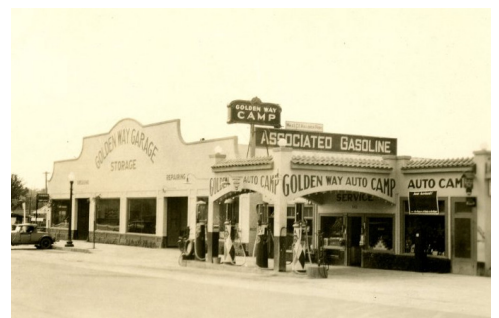
Golden Way Garage and service station, along El Camino Real (Atascadero Historical Society, 1969).
