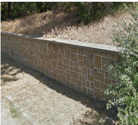
Stone masonry wall (Chung, 2018).
