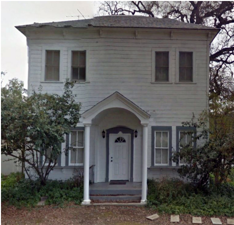
Henry Ranch House, with symmetrical facade and elaborate entry (Chung, 2018).
