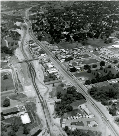
Construction of the new US 101 lanes, to the left, with the original alignment seen to the right (Atascadero Historical Society, 1955).
