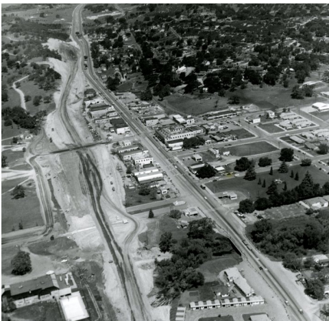
Highway 101 construction (Atascadero Historical Society, 1955).
