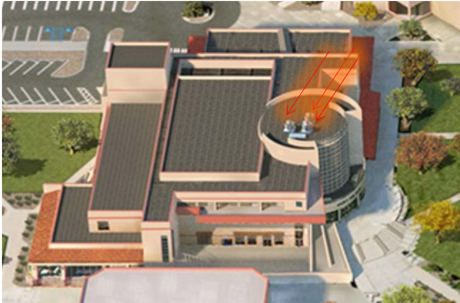
Figure 7-4 - Roof Mounted Exhaust Fans
