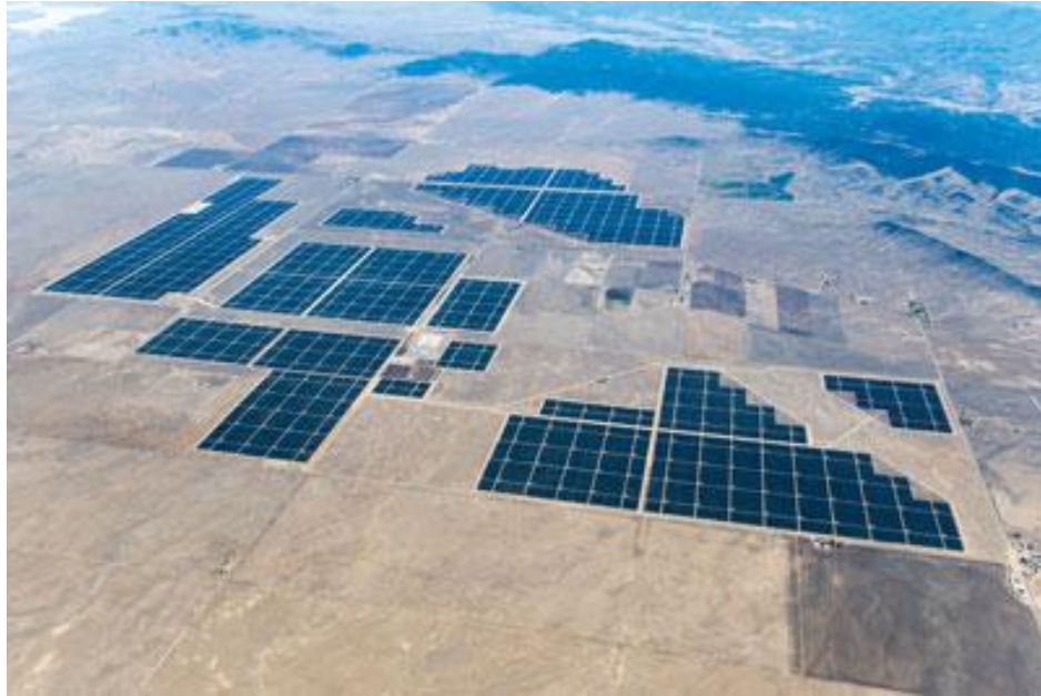
Figure 1-1. Topaz solar farm [5].
