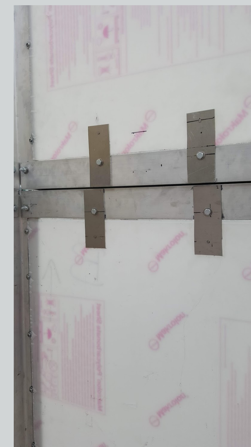
Figure 8: The four metal plates provide support to keep the Plexiglas from moving inward and possibly breaking
