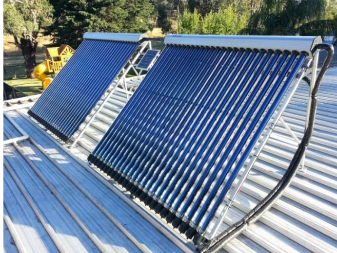
Figure 3.4: Solar Water Heater Collector System [29]
