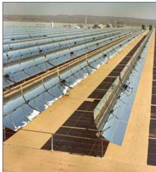
Figure 2.13: Parabolic Trough System Array [12]
