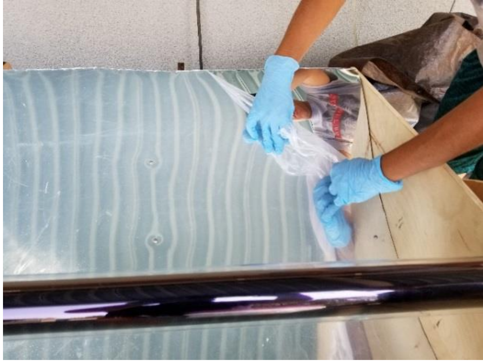
Figure 3.27: Removal of ReflecTech® Protective Liner
