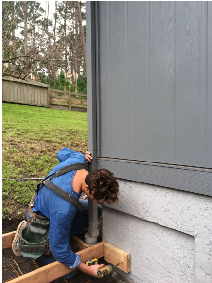
Fig. 1: 2x6 block connection.
