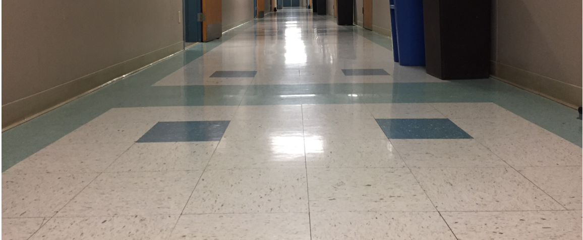
Figure 4.8: The Lower Half of the Electrical Engineering Hallway
