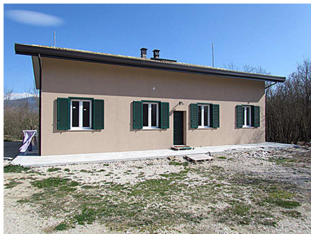
Fig. 9. Off-grid residential house.
