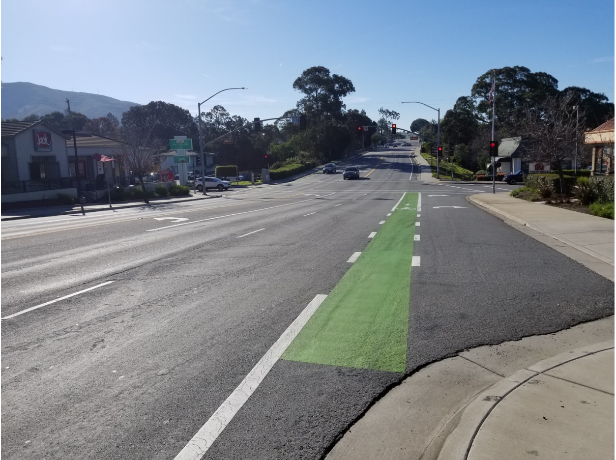
Figure 6: Class II bikeway painted in green to standout on SR 1 in San Luis Obispo
