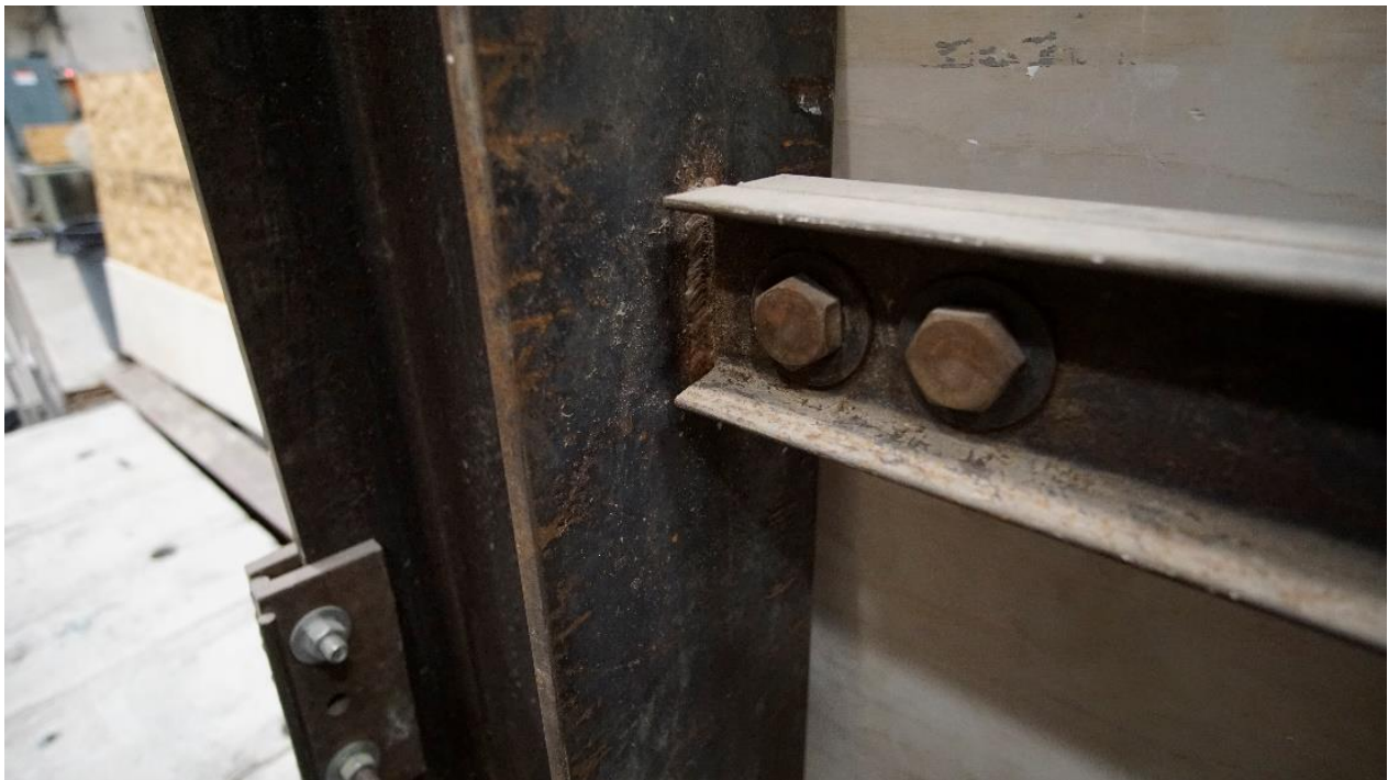
Figure 21 : Intermediate Horizontal Member for Main Brace
