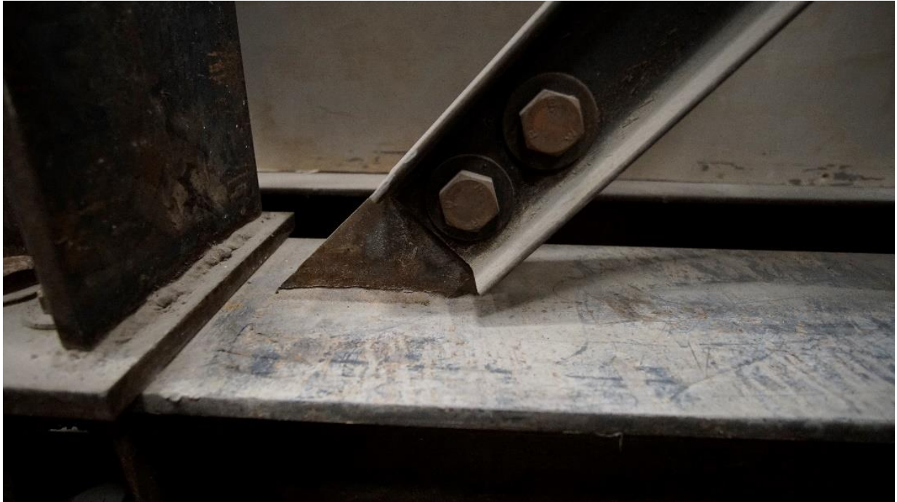
Figure 22 : Intermediate Diagonal Member for Main Brace
