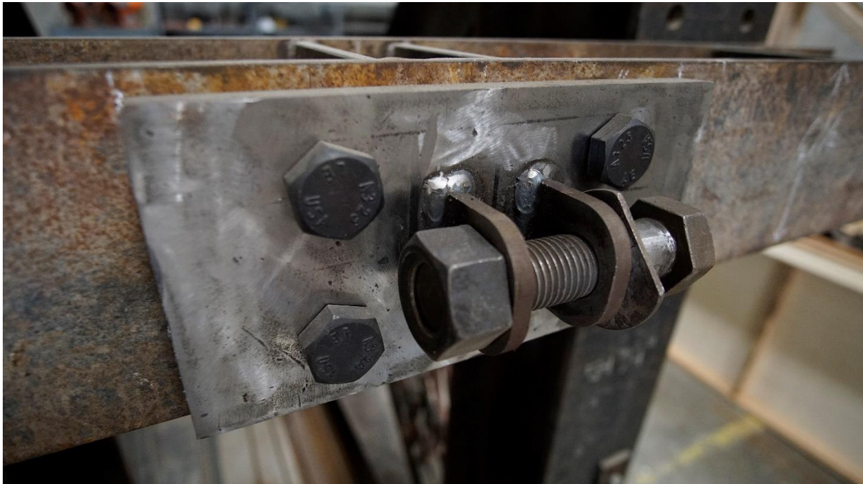
Figure 16 : Sandwich Plate on Horizontal Beam
