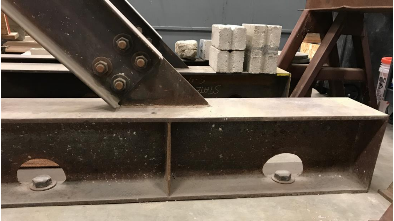
Figure 24 : Brace to Floor Beam Connection
