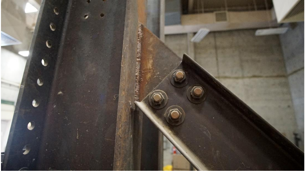
Figure 20 : Brace Connected to Column with Gusset Plate
