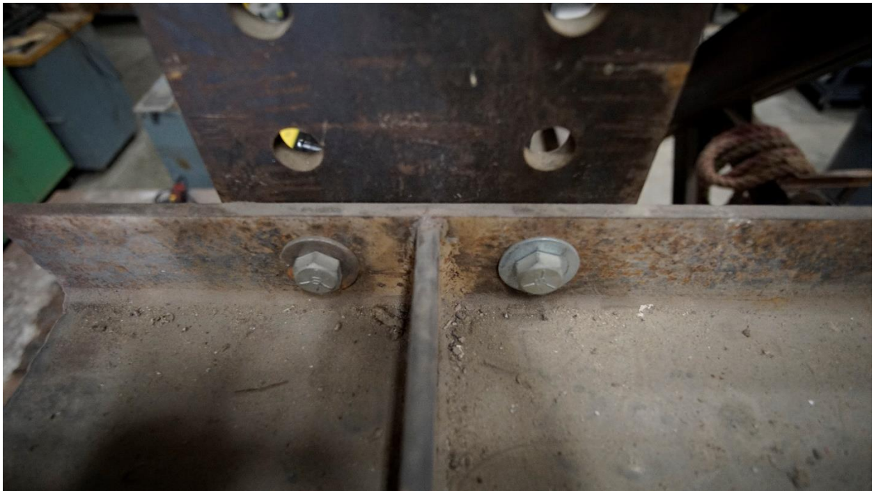
Figure 18 : Stiffener Plate in Horizontal Beam
