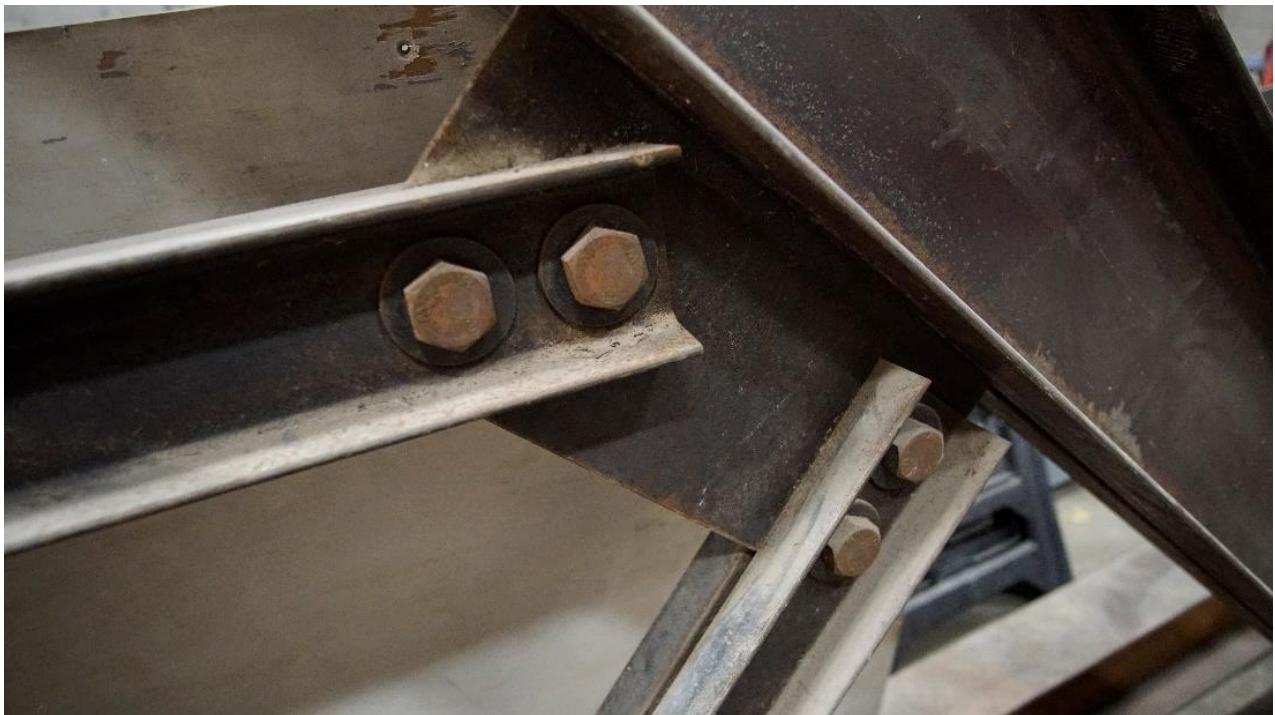
Figure 23 : Main Brace Gusset Plates Bolted to Intermediate Members
