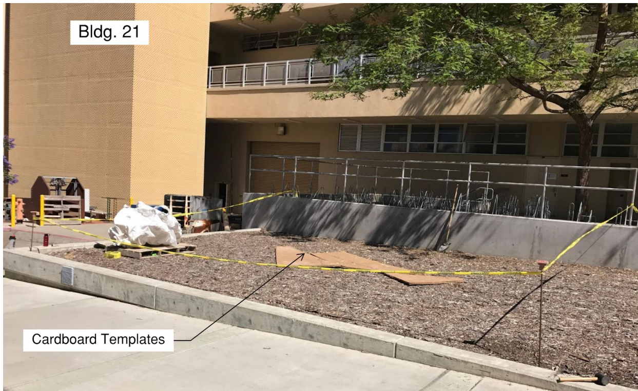
Figure 13: Base and Spacer Plate Templates Oriented on Site with Construction Fence
