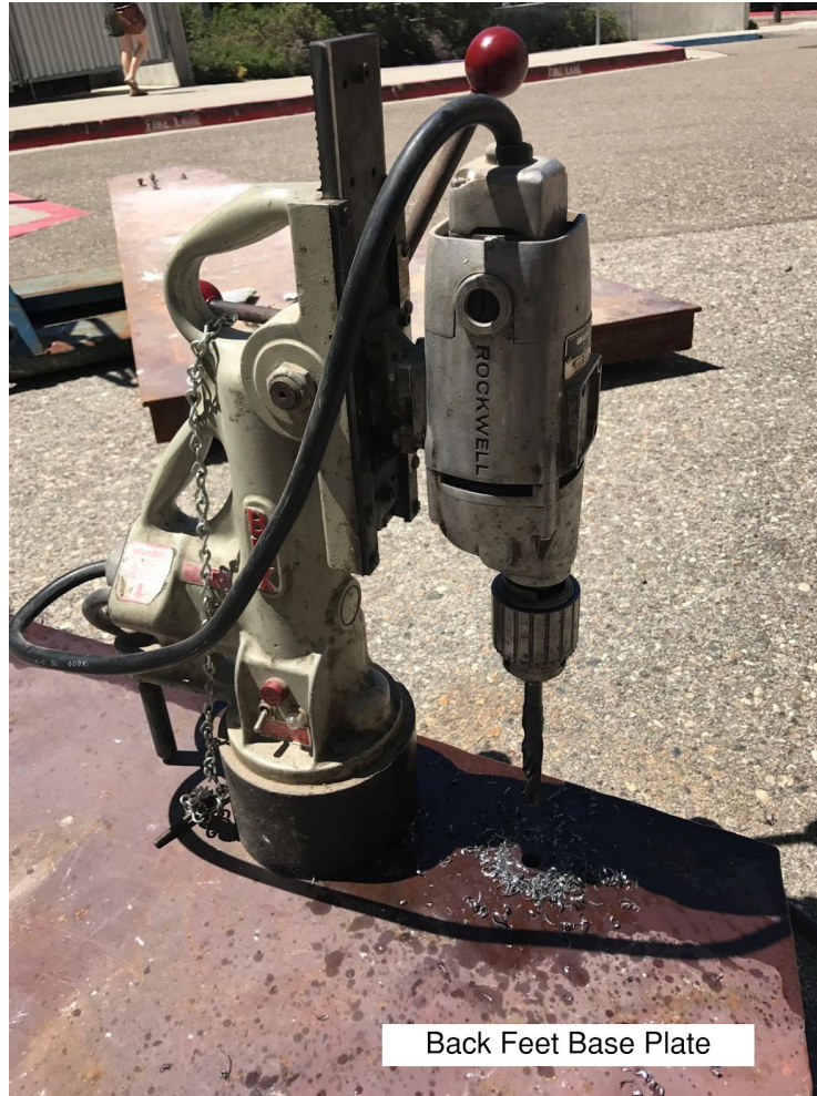
Figure 18: Mag Drilling Hole in Base Plate
