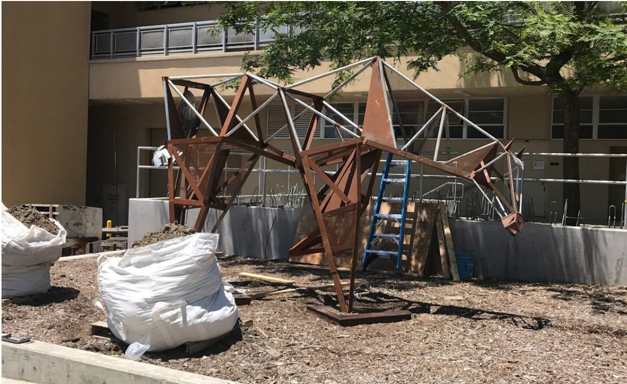
Figure 21: Fully Erected Sculpture
