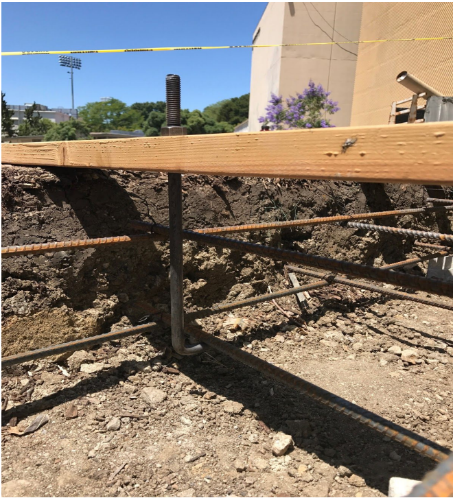
Figure 15: Rebar Cage and Anchor Bolt Positioned in Excavation
