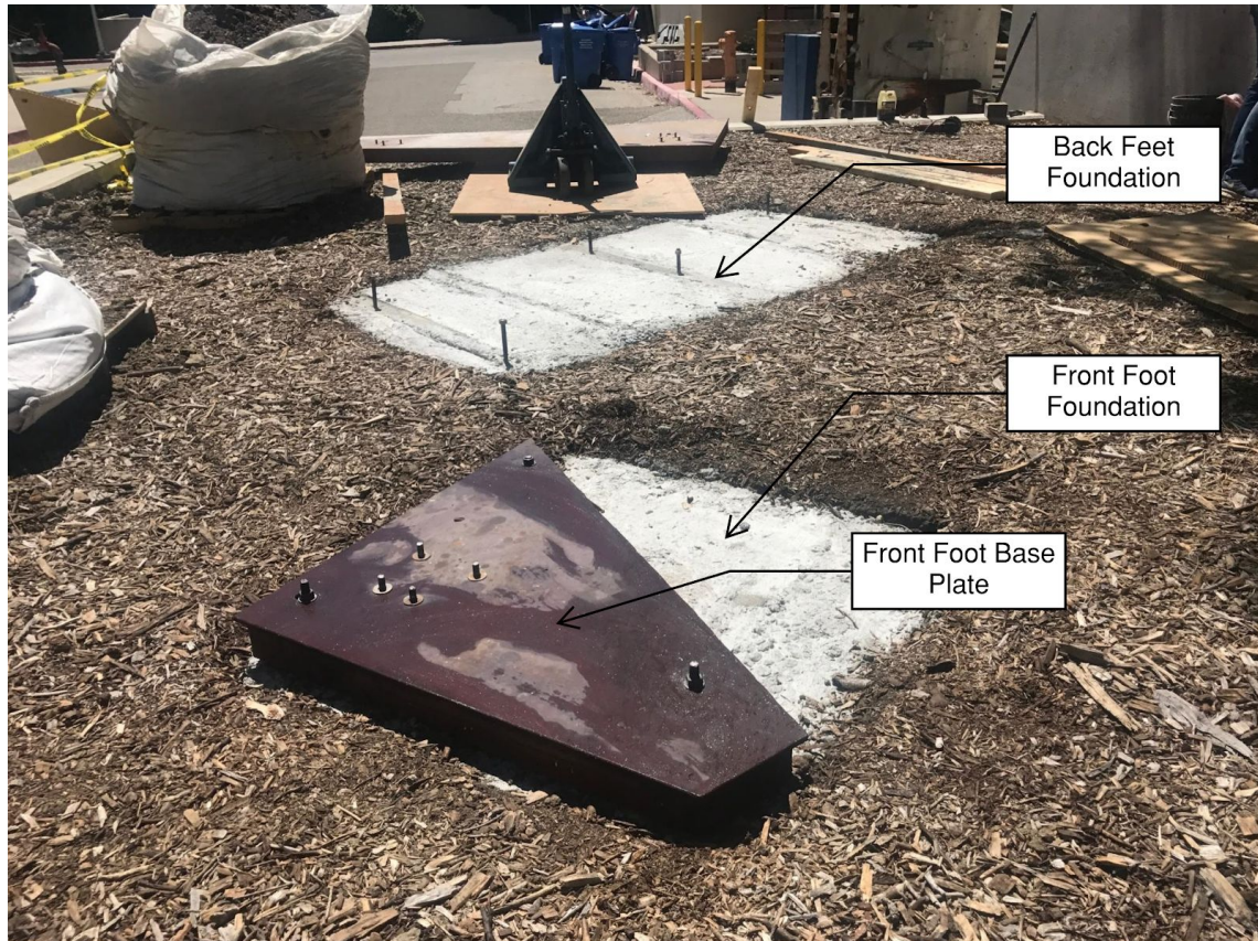
Figure 19: Base Plate on Foundation
