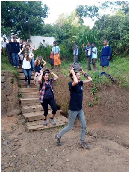
Students carrying rocks for retaining wall in Sunzu Village
