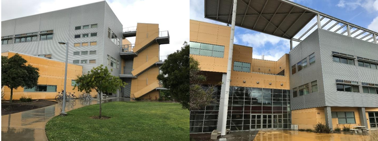
Figure 2. East entrance to Engineering IV. Stair #4 is shown as one of the three exterior exit stairways serving the building. (left) The main entrance to Engineering IV leads into a three-story atrium space with a communicating stair. (right)
