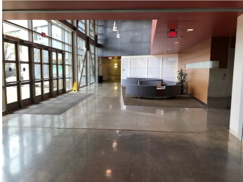
Figure 26. Sofa arrangement in the first-floor lobby area. Two spot-type photoelectric smoke detectors can be seen under the balcony at the top-right.
