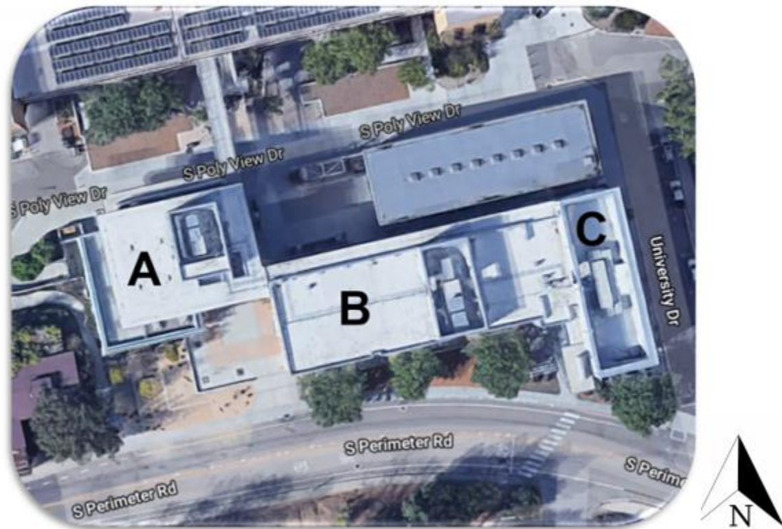
Figure 2: Aerial View of The Construction Innovation Center
