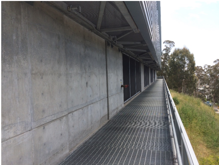
Figure 33: West Side Exterior Walkway and Hose Outlet
