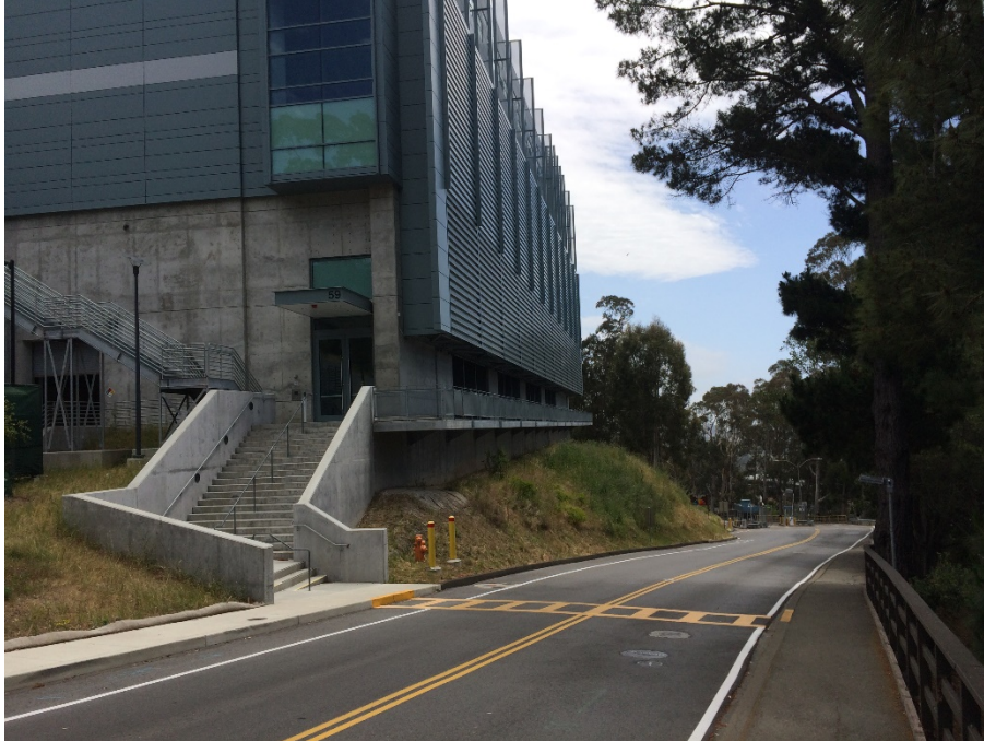
Figure 32: West Side Building Limited Access
