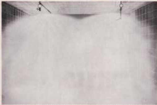
"Automatic" SPRAY Sprinklers discharging water at moderate pressures provide good lateral and downward coverage.
