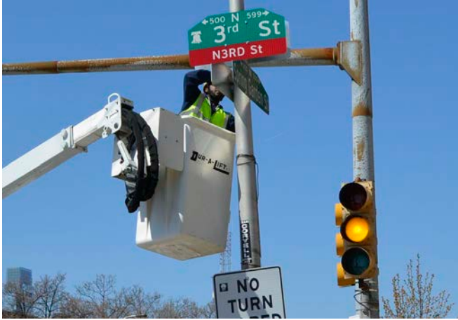
Figure 22: N3RD Street Sign (Levesque 2014)
