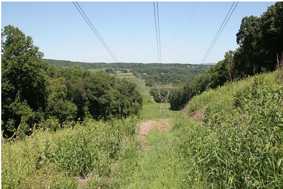
Powerline right-of-way, view north from the forested slope at the southern end of the property
