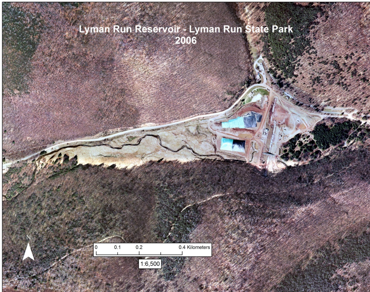
Figure 3 - Lyman Run Lake dam under construction; 2006
