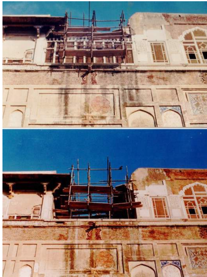
Figure 22: Repair by disassembly of the marble jalis (2000).
