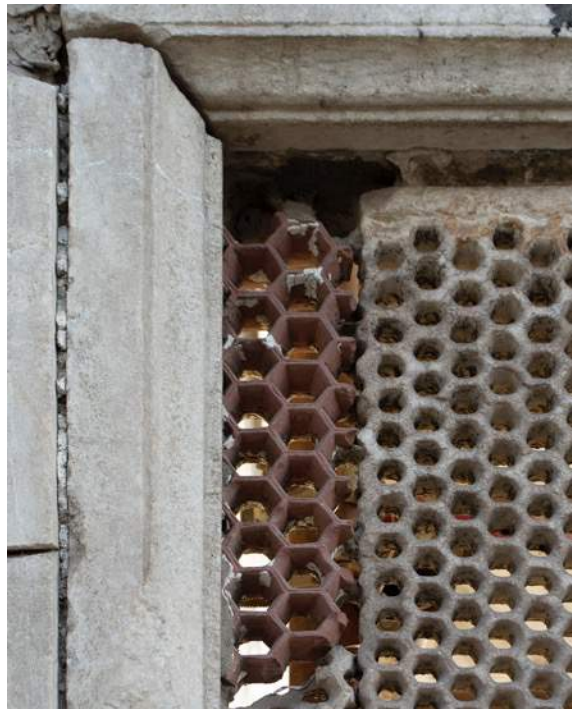
Figure 37: Dutchman repair of the marble jali with terracotta.
