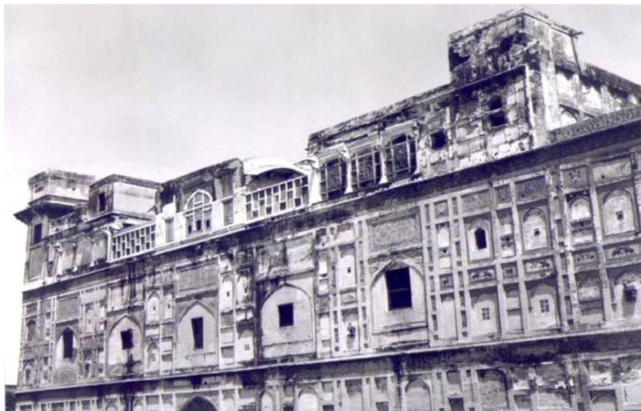
Figure 20: Historical photograph of the western façade of Naulakha (ca. 1900). Showing the missing western chajja (eave) in relation to the rest of the roof.
