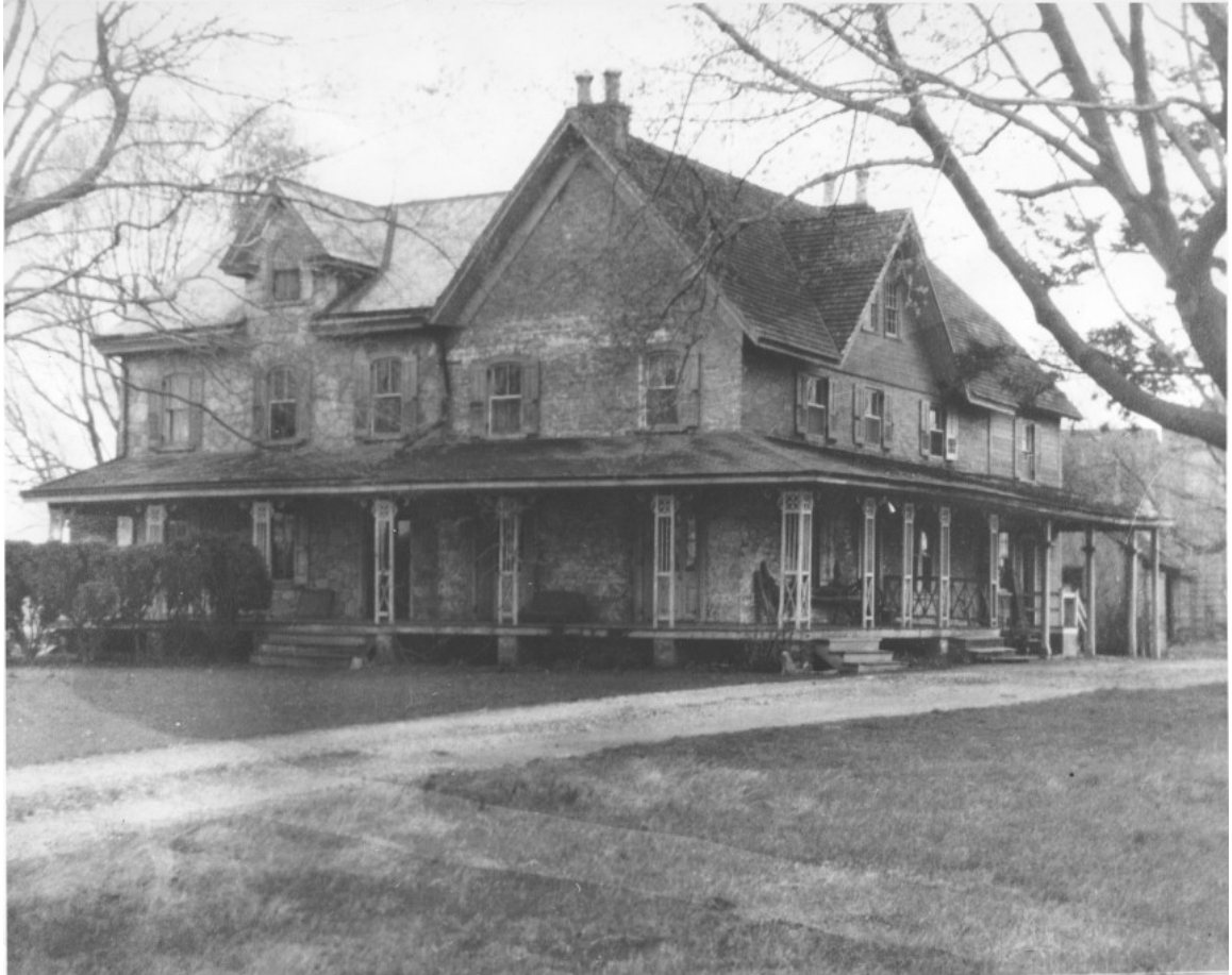
FIGURE 12: West elevation of the 1704 House in 1953 showing signs of general disrepair. (Image: Clement S. Brinton, 1953 from Photo Archives, Chester County Historical Society Library)
