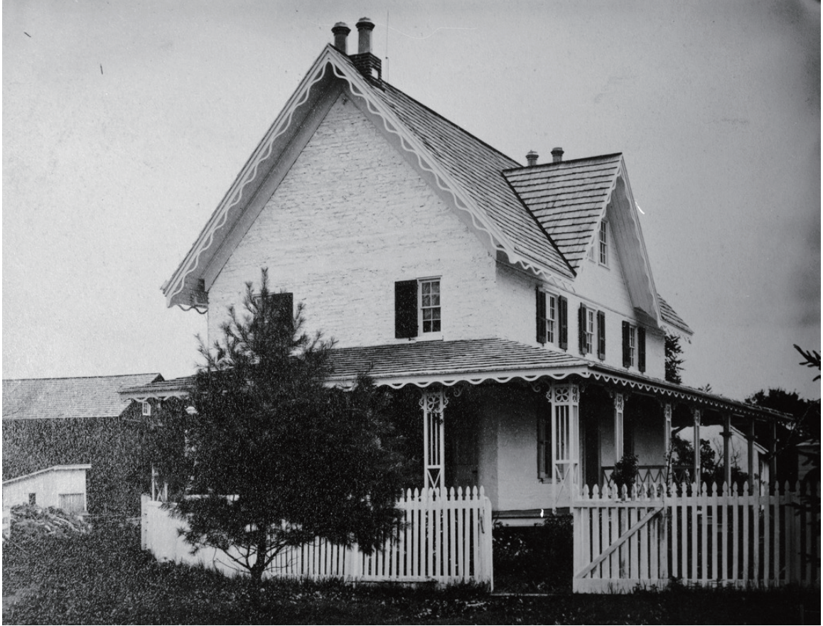
FIGURE 6: West elevation of the 1704 House ca. 1870 showing the modifications completed by Ziba Darlington, and early modifications by Henry Faucett (gable dormers and wrapped porch) (Image: T.W. Taylor ca. 1870, from the Photo Archives, Chester County Historical Society).
