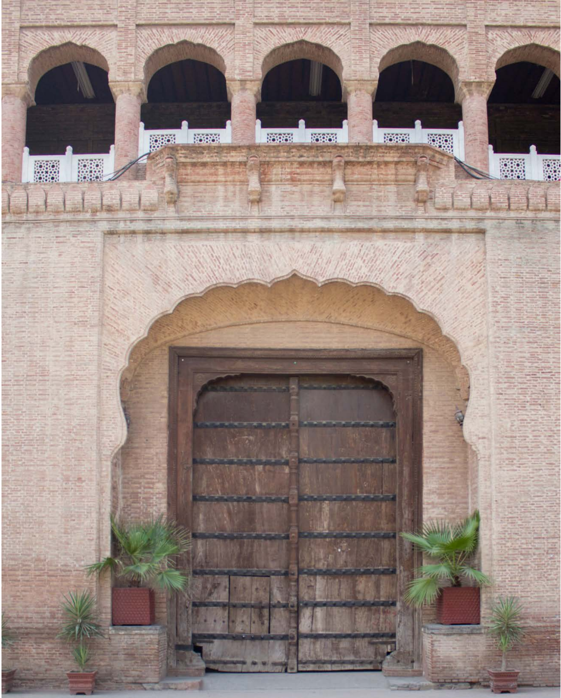
Fig. 41: Historical Door of Khushal Singh Haveli still in use. The upper story shows arcaded areas, verandahs that facilitate in ventilation and visual connectivity (Source: Awais Jibran)
