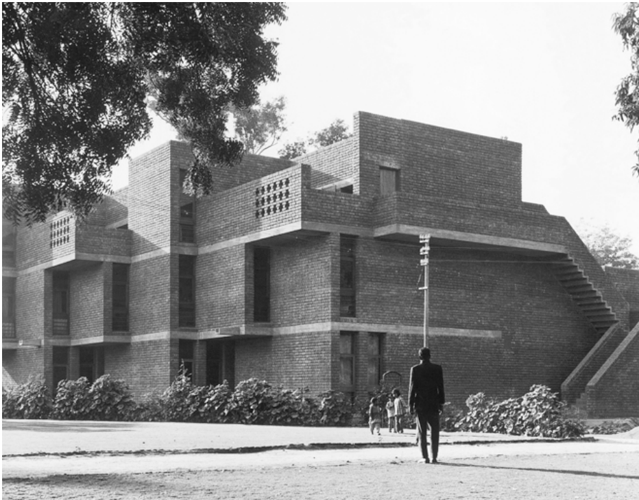
Fig. 49: Western Facade of French Embassy Housing. (Source: Rajrewal.in)
