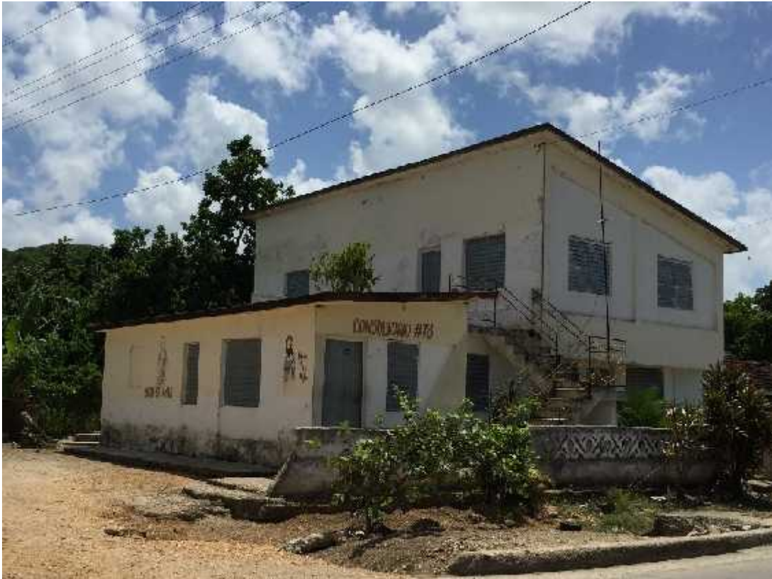
Figure 1: Two-floored structure of a CMF that serves both Mayajigua and nearby Chambas. Photo was taken in 2016 by Ivana Kohut.
