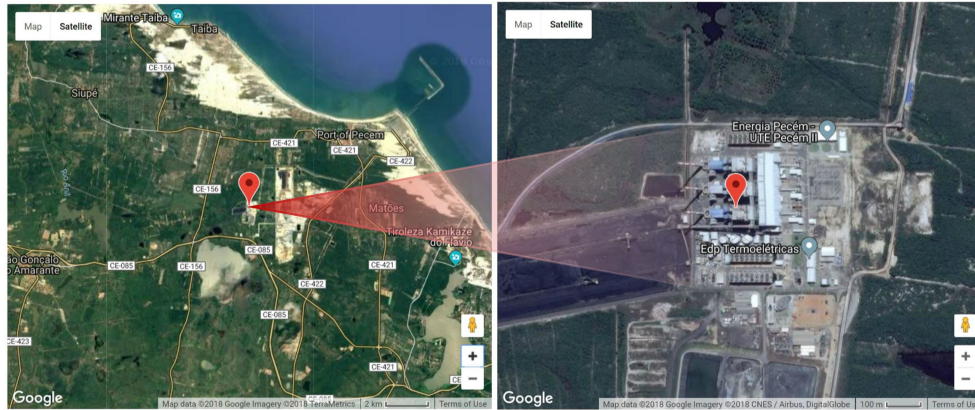
Figure 7.2: Satellite images of the Porto Do Pecem Power Station in Ceara, Brazil. Obtained using Google Maps.
