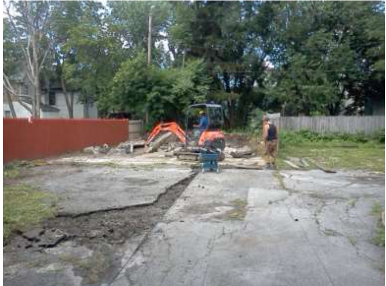
De-paving a vacant lot to implement a rain garden
