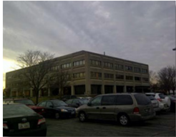
Office building in which Gordin Medical leased one of its medical suites
