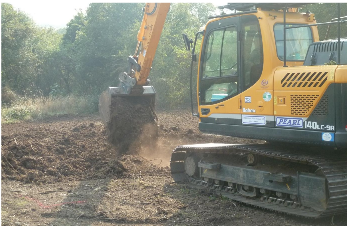
Figure 11. Soil inversion subplot being created at Hadleigh Park, September 2016.
