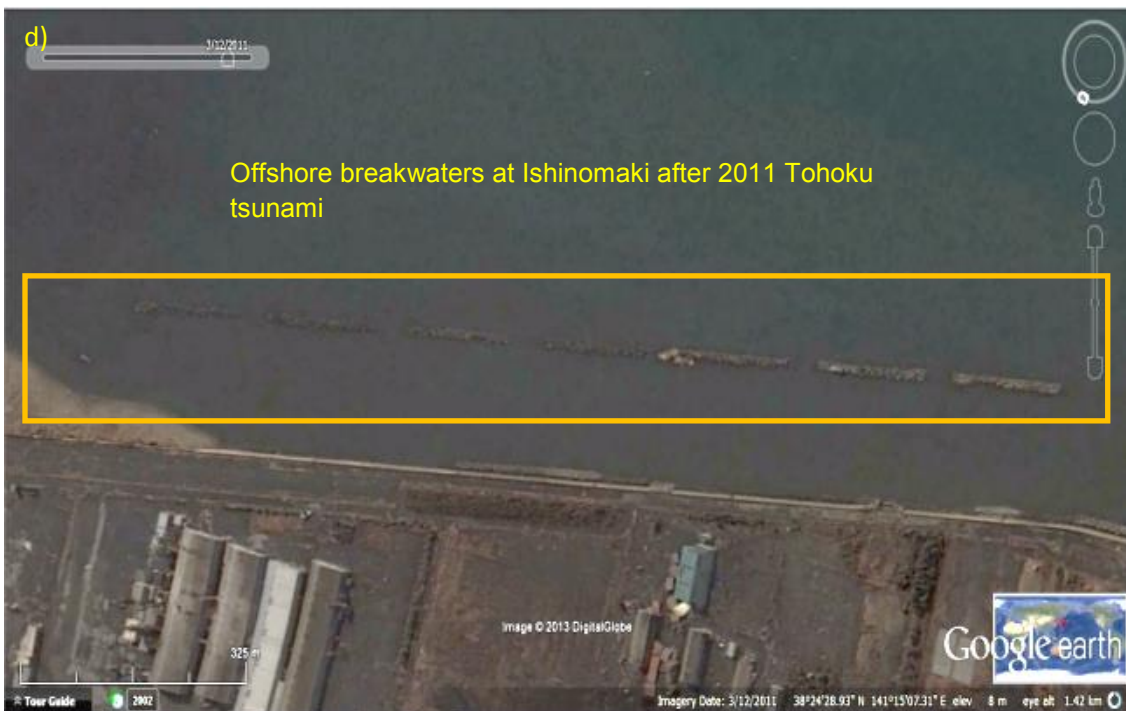
Figure 9. Breakwater failure: a) Offshore breakwater failure at Watari (North), b) Offshore breakwater failure at Ishinomaki (East), c) and d) Offshore breakwaters at Ishinomaki before and after 2011 Tohoku tsunami (Image Source: Google Earth).
