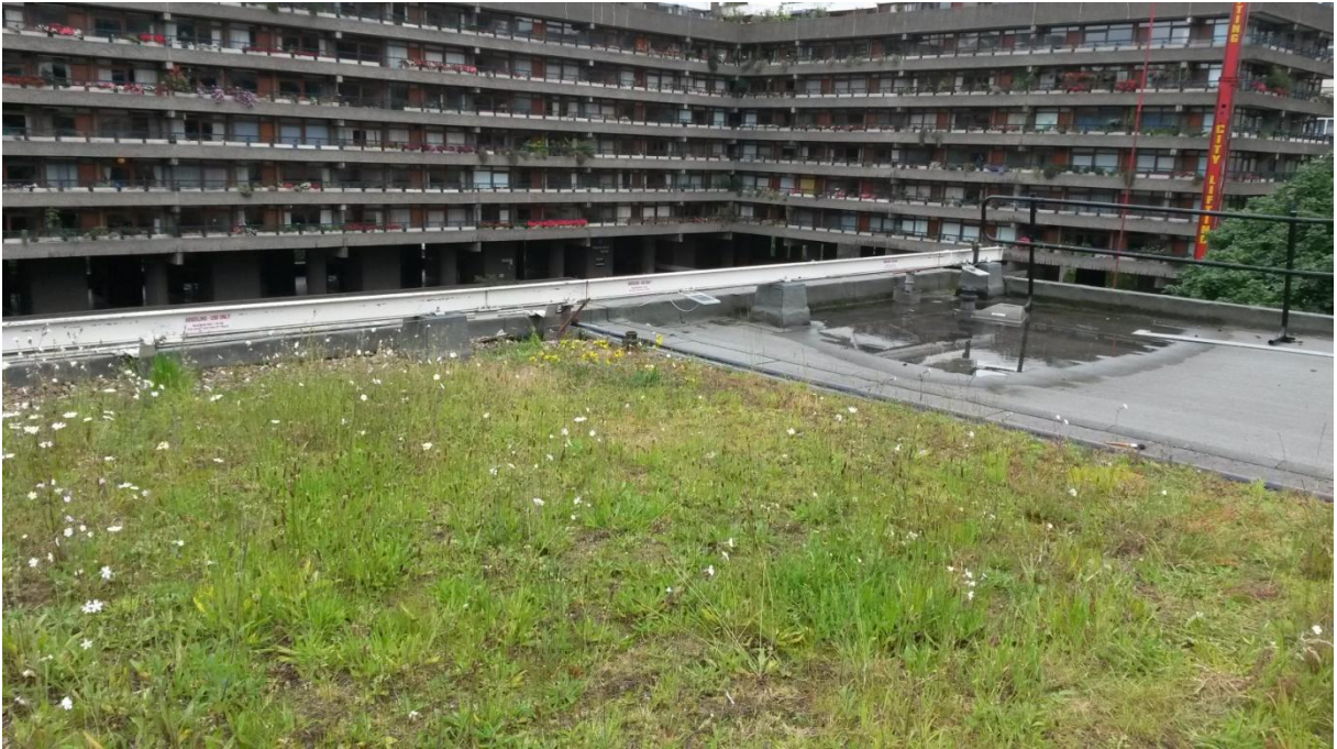
Figure 3. Installed green roof on the northwest corner of the Museum of London roof.
