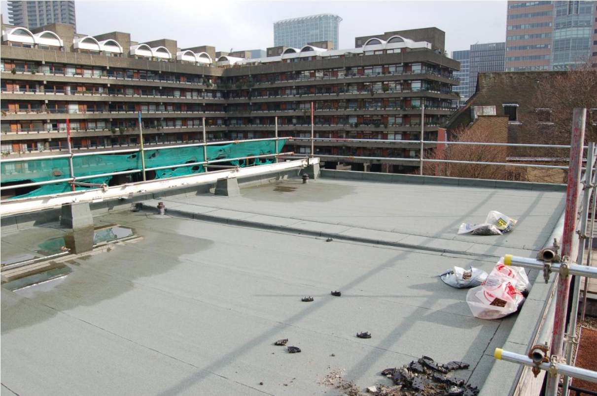
Figure 2. Area of the Museum of London roof to be greened.
