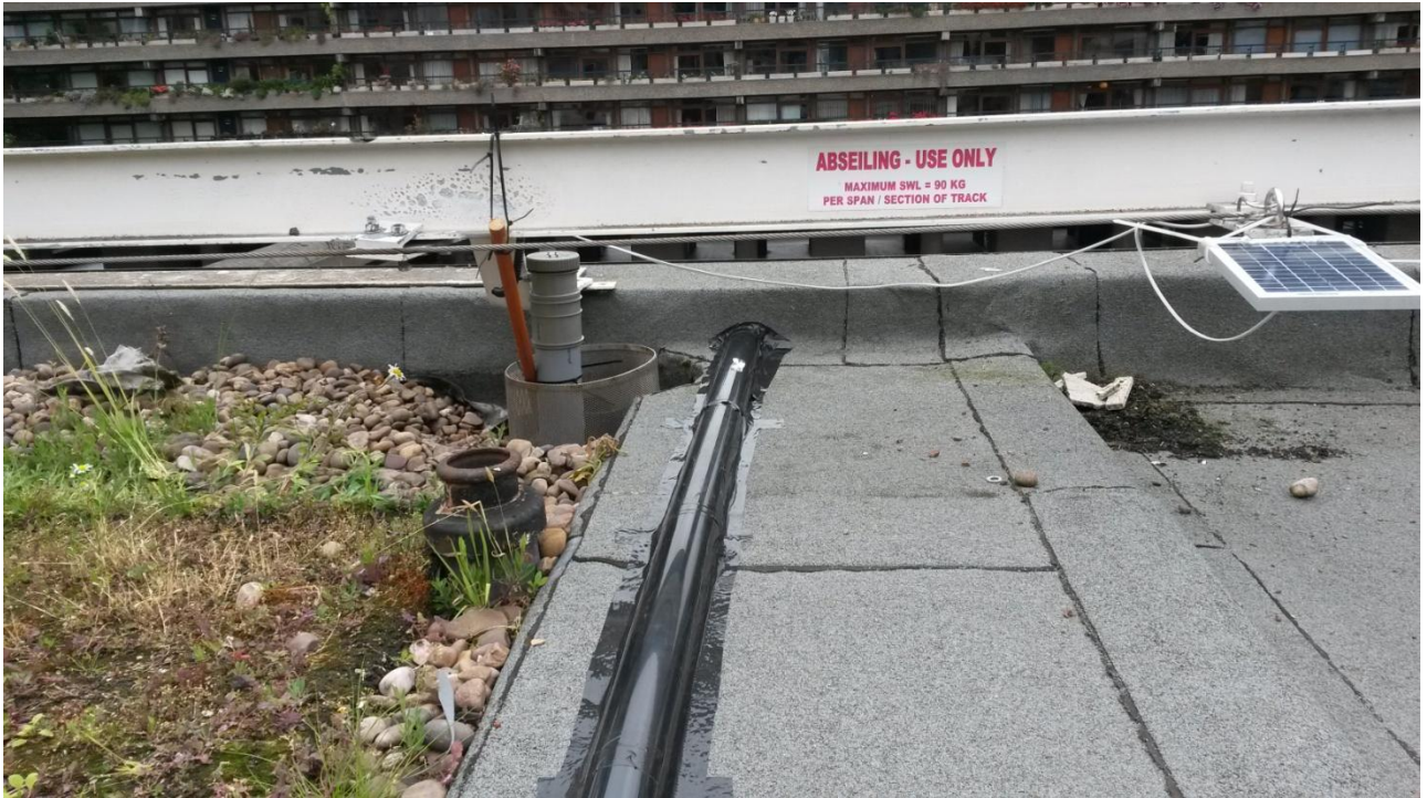
Figure 7. Barrier dividing the green roof catchment from the control roof catchment.
