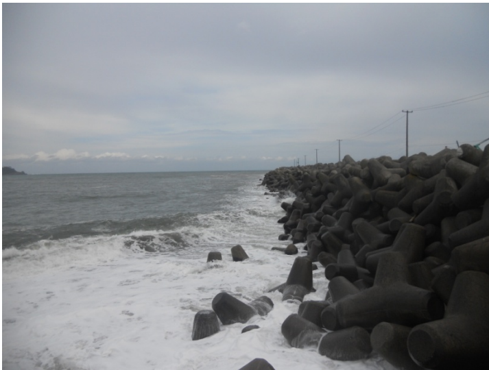
Figure 4. Steep Tetrapod Armour Layer at Kuji Port.
