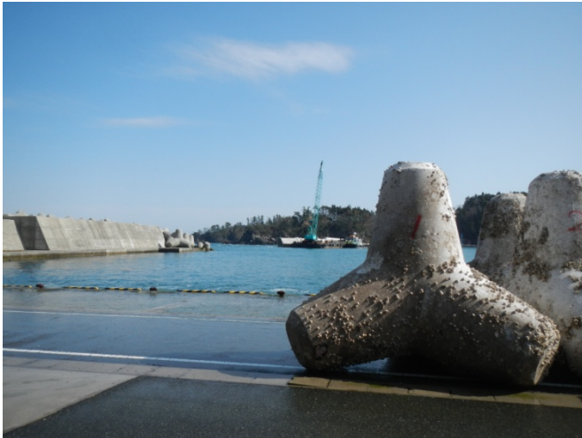
Figure 8. Recovered tetrapod units at Ishimaha port were temporarily stored behind the breakwater before being placed back in their original location
