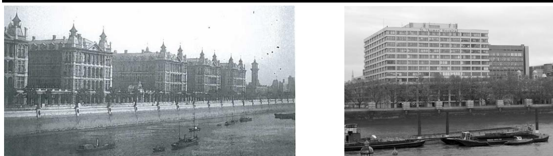
Left: Appendix F.26 Photograph of South Wing, St. Thomas' Hospital before the World War II bombing (Guys and St. Thomas' Capital Estate & Facilities Department). Right: Appendix F.26a 2012, Photograph of North Wing, St. Thomas' Hospital.
