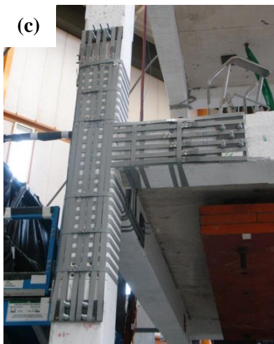
Fig. 11. PTMS strengthening of beam-column joints: (a) fixing of steel plates, (b) additional anchorage plate at interior face of beams, (c) final view of 1 st floor joints, (d) final view of 2 nd floor joints.
