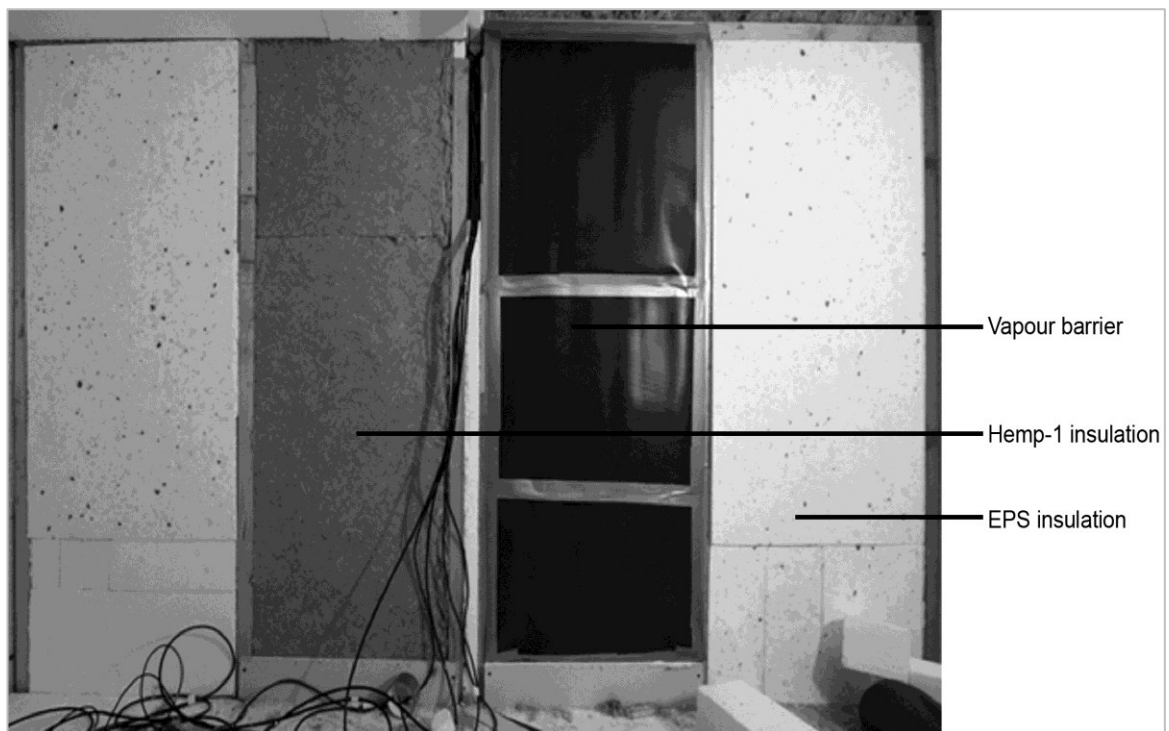
Figure 7.13: The installation of the outer layer of the insulation.
