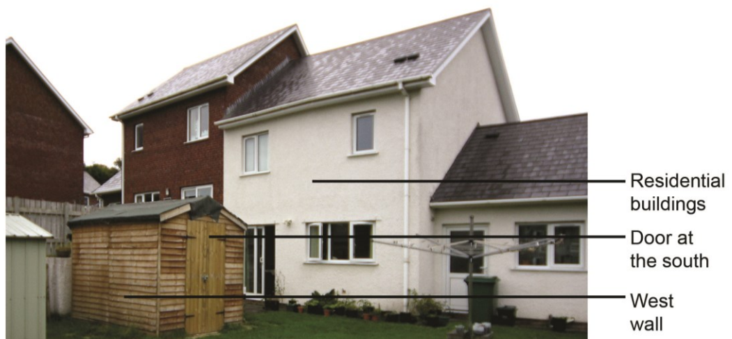
D.3: Illustration showing the test building and the residential buildings at the east side of the test building.
