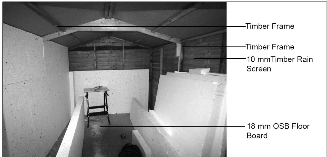
Figure 7.4: Construction of the outer layer of the test building.
