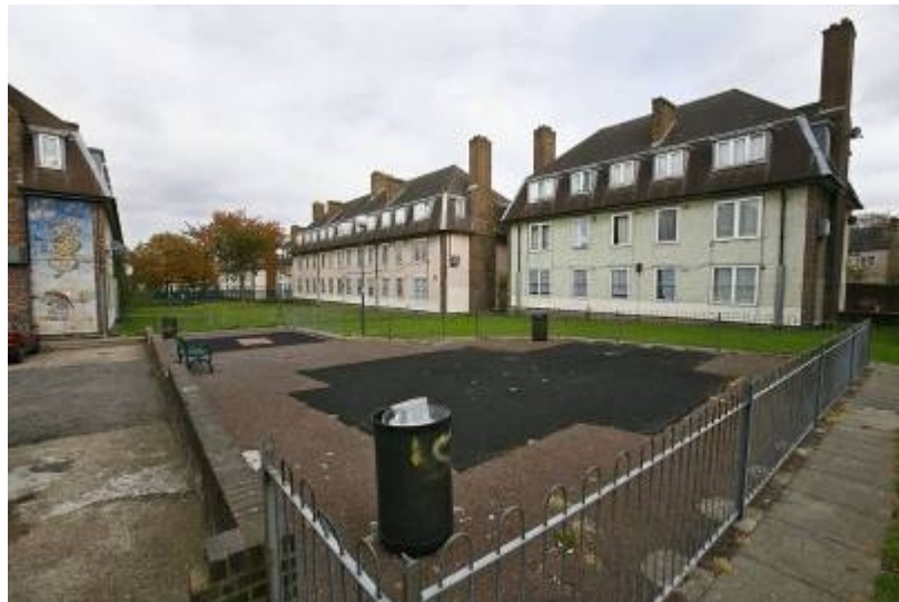
Picture 6.1 – WL intervention area (I)
