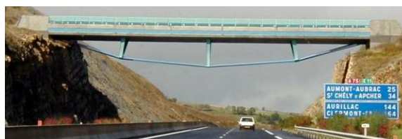
Figure 3. Truc de la Fare fauna overpass (photograph courtesy of Nicholas Janberg, www.structurae.de )
