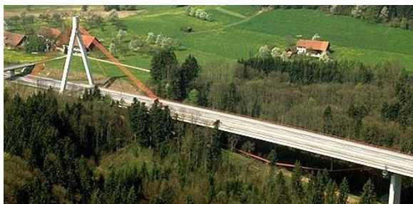
Figure 2. Obere Argen Viaduct (photograph courtesy of Jorg Schlaich, copyright Elsner, Gert, Stuttgart).
