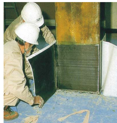
Fig. 1 FRP confinement of concrete columns
