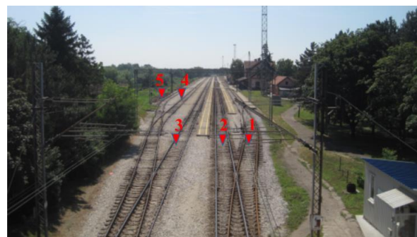
Fig.1. Pančevo Varoš railway station
