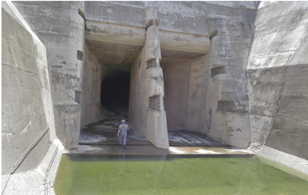
Figure 2. FP-BA tunnel entrance building
