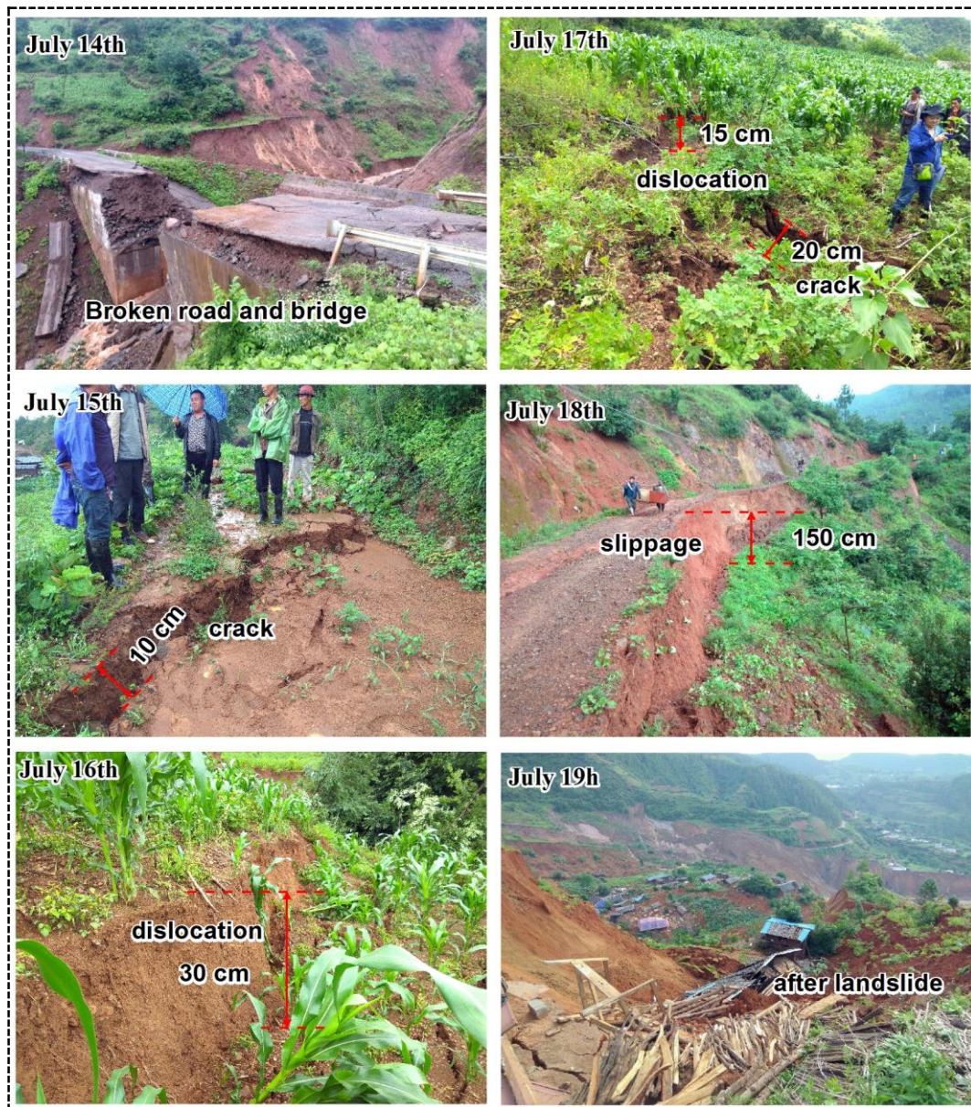
Fig.5 Deformation characteristics of the Boli landslide from July 14th to 19th
