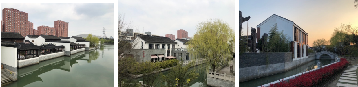
Figure 8. View of New Building Area
