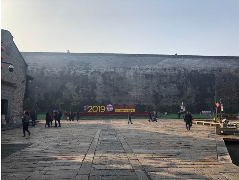
Figure 26. The section of City Wall in Laomendong Historic District
