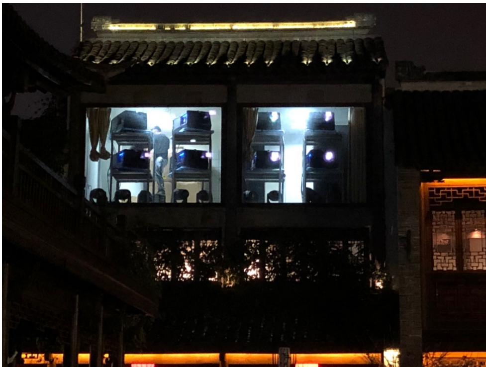
Figure 32. 3D mapping projectors and lights
