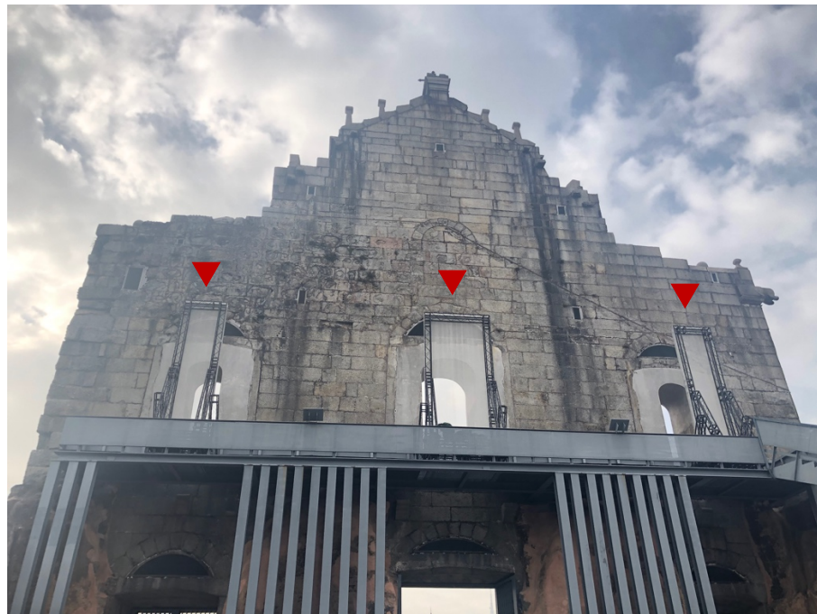
Figure 44. Screens for filling the holes on the facade
