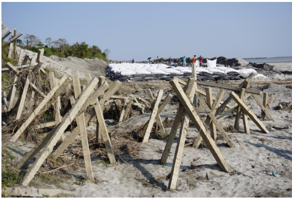
Figures 39-40: R.C.C Porcupines constructed by the Brahmaputra Board.
