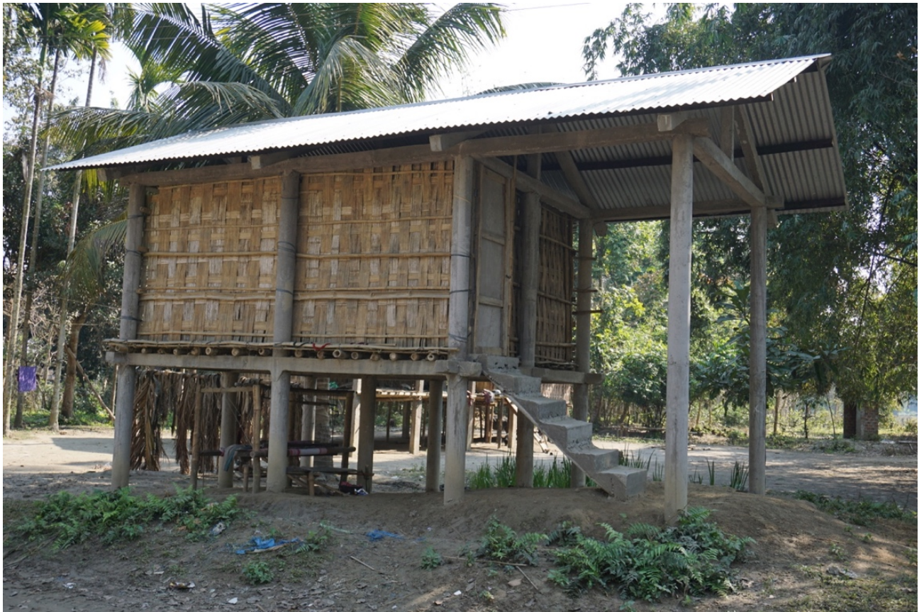
Figure 36: Traditional Mishing house with concrete stilts and structural members, Thatch roof is also replaced by tin roof.
