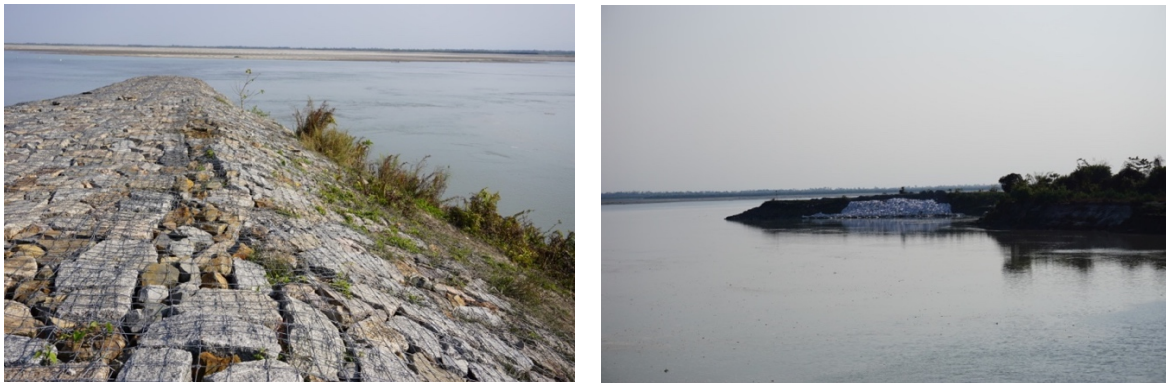
Figures 41-42: Land spurs constructed by the Brahmaputra Board.
