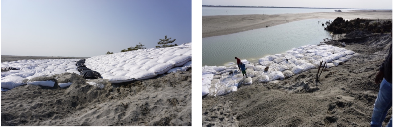
Figures 43-44: Bank Revetment construction by Brahmaputra Board.
