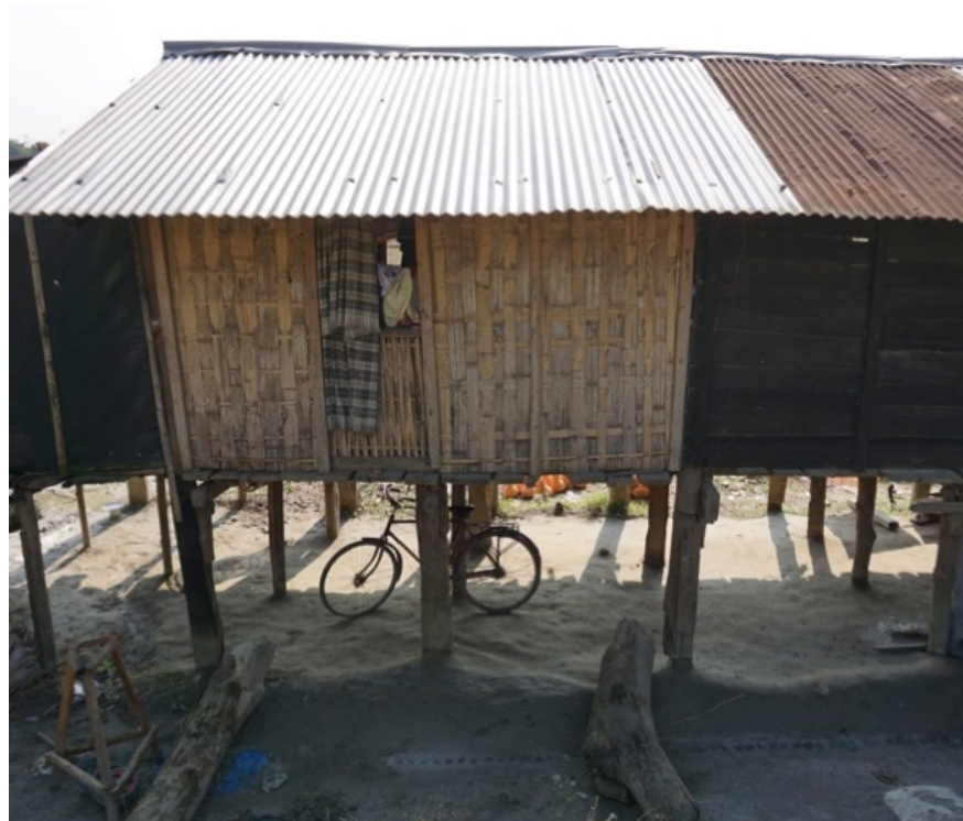
Figure 12: Wattle and daub construction with wood panels and tin roof.
