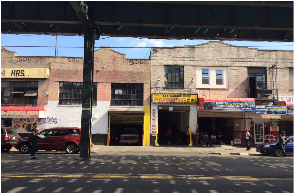
Figure 33: Historic garage structures on Jerome Avenue. https://www.documentcloud.org/documents/3943782-DCP-s-Presentation-to-CPC.html .
