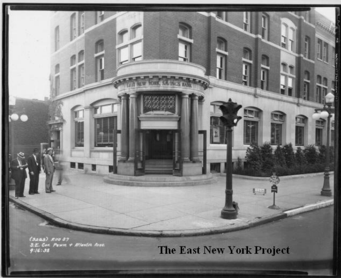
Figure 9: East New York Savings Bank (demolished), The East New York Project, http://www.tapesare.com/Penn.html .
