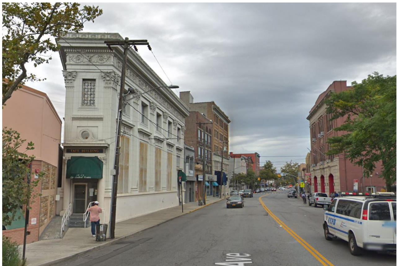
Figure 21: Ornamented Terra Cotta building across from Firehouse. Google StreetView.
