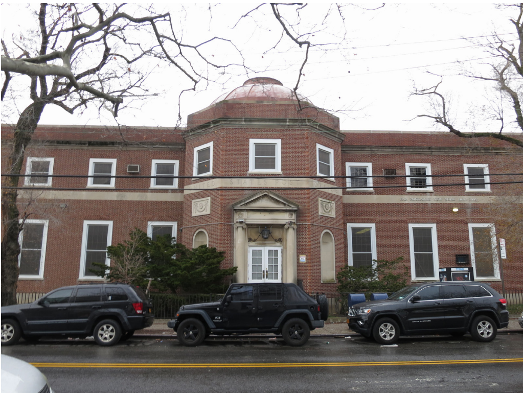
Figure 17: Far Rockaway Post Office, listed on the State and National Registers. From Chapter 7, FEIS.
