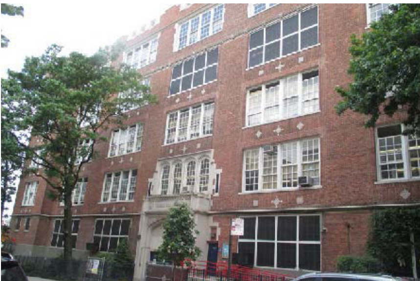
Figure 37: P.S. 98, found to be eligible for both State and National Register listing. From Chapter 7, FEIS.
