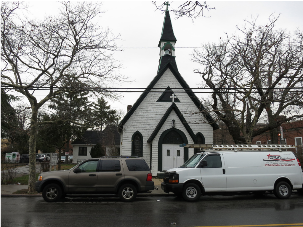
Figure 16: Trinity Chapel, listed on the State and National Registers. From Chapter 7, FEIS.
