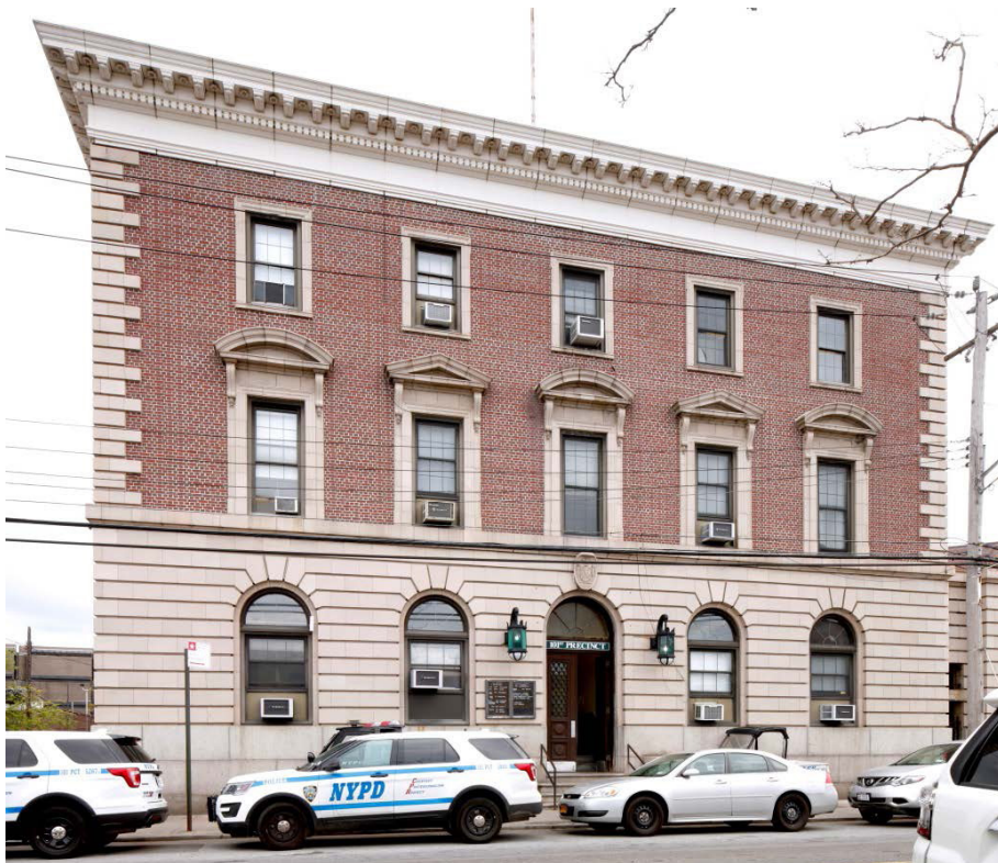
Figure 19: The 53rd (now 101st) Precinct Police Station at 16-12 Mott Avenue, Far Rockaway (1927-28).
