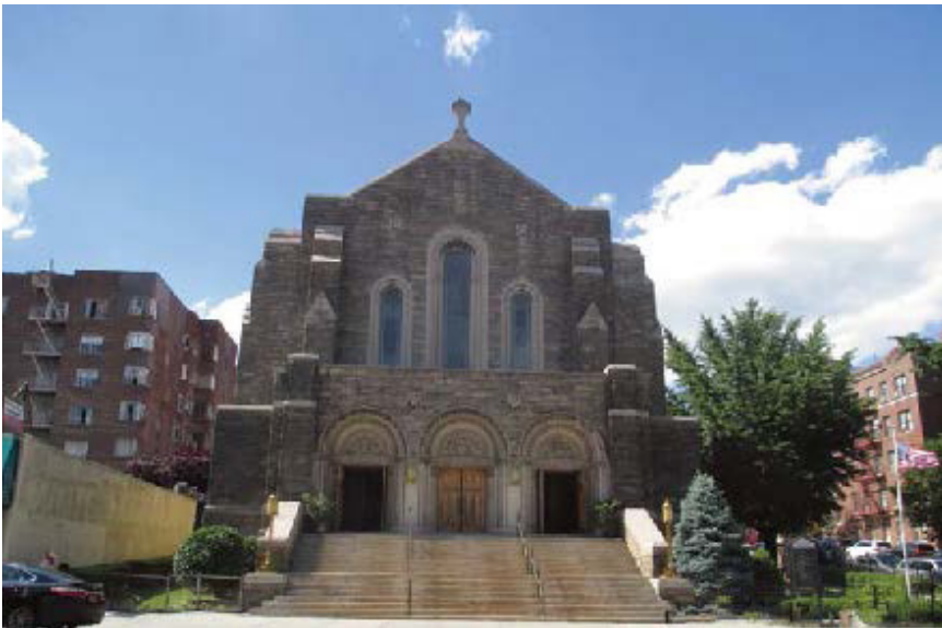
Figure 35: The stained glass windows of Good Shepherd Roman Catholic Church could be adversely affected by nearby construction. From Chapter 7, FEIS.
