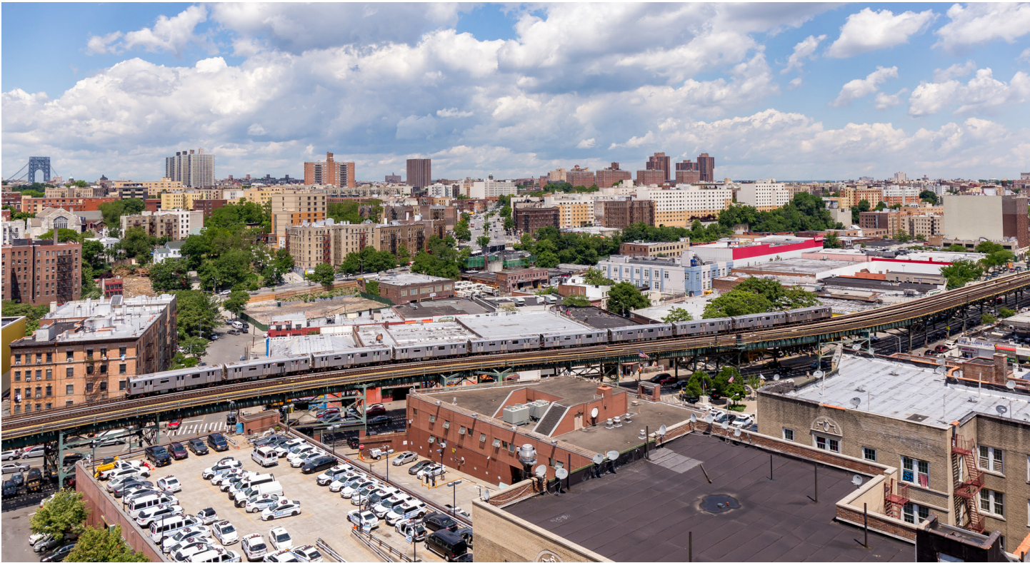
Figure 29: Context photo of Jerome Avenue and the elevated 4 train. https://citylimits.org/2016/11/25/jerome-avenue-photo-essay/ .
