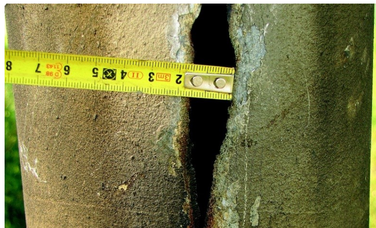
Obr. 2.2 - 3 – Trhlina [8]
