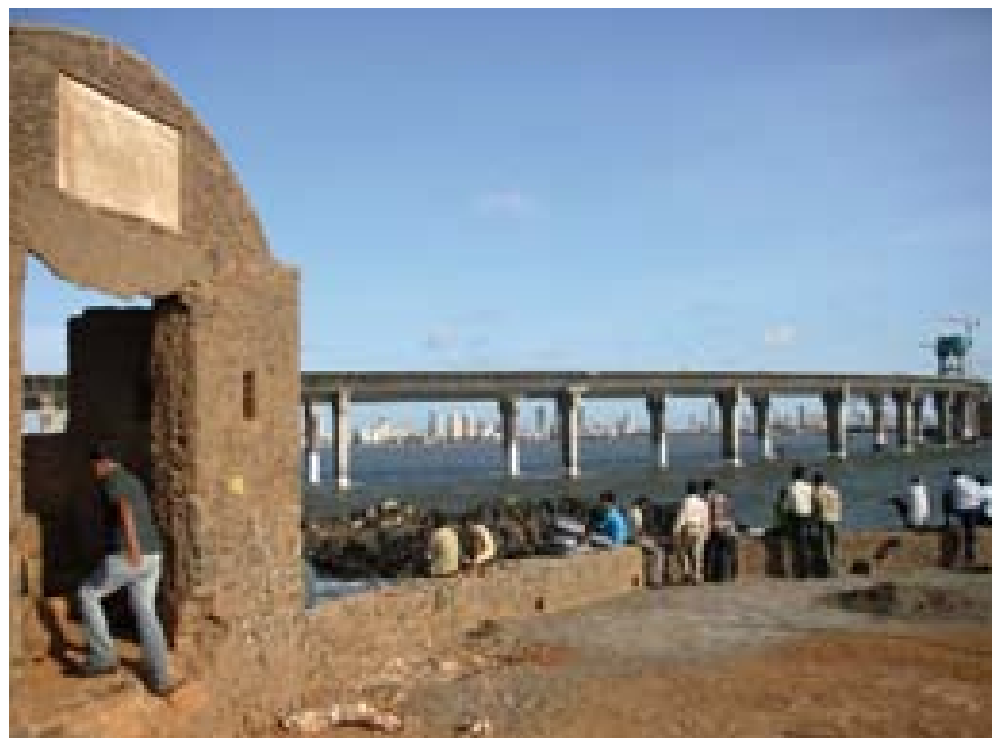
The Bandra-Worli sea link forms part of the Western Express Highway.
