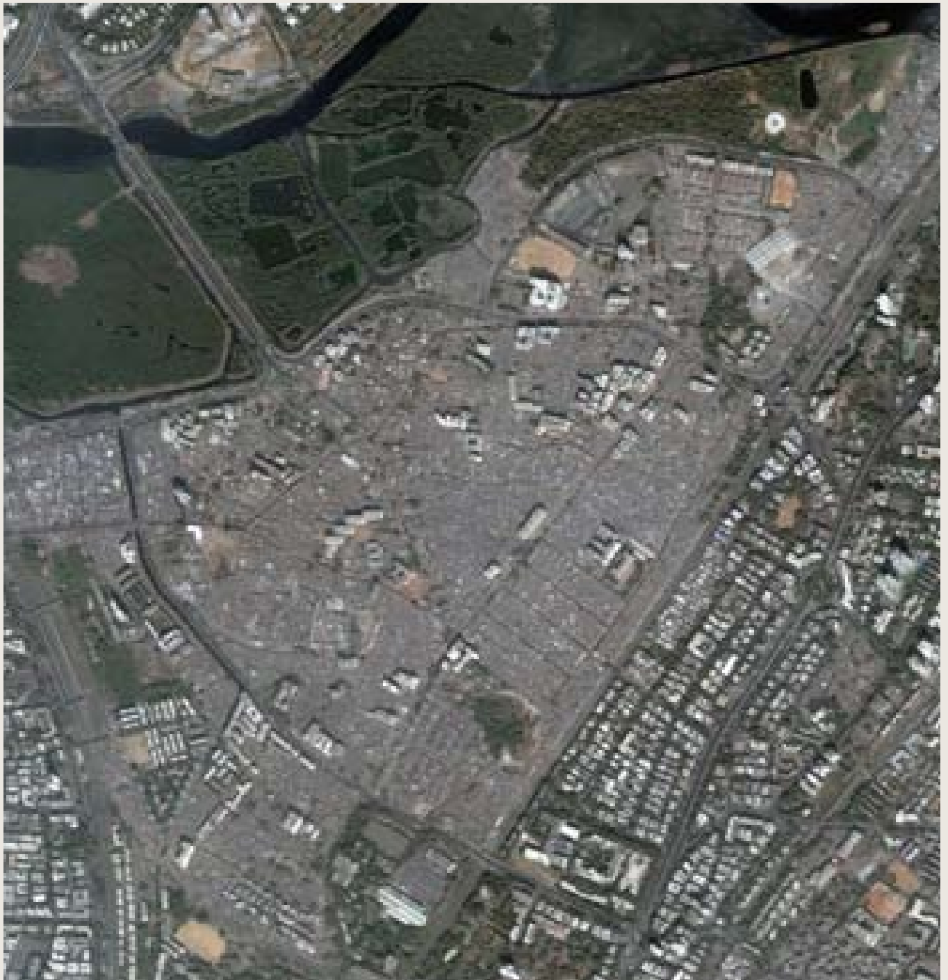
This aerial view of Dharavi (1:11,500) captures the fine grain density of the area's 2.36 km 2 (583 acres) and location in the heart of Mumbai, surrounded by multiple transport routes and middle income suburbs.
