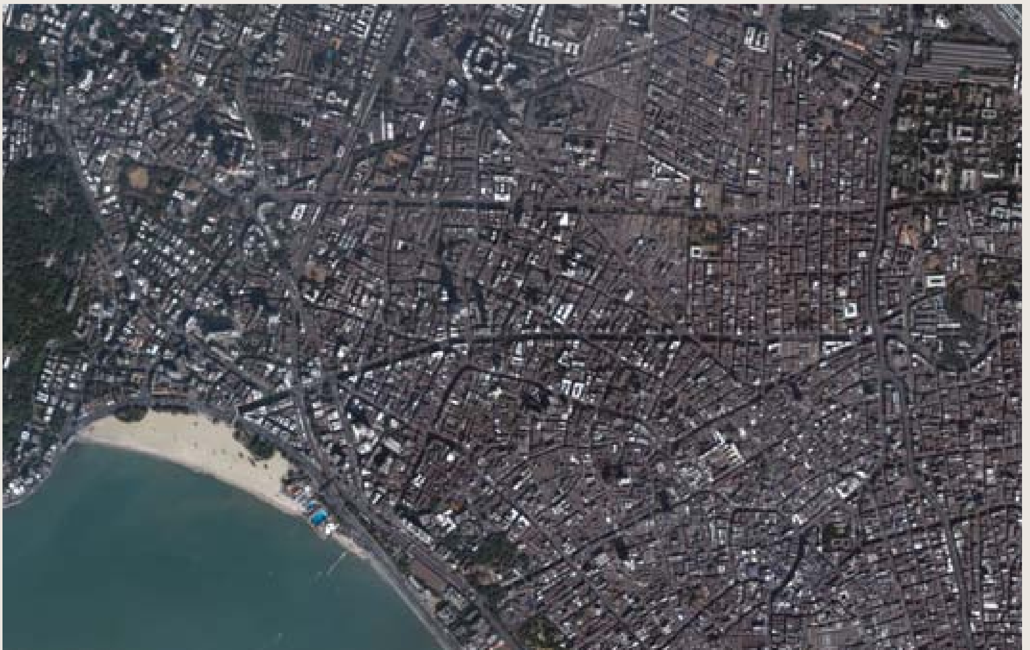
With an average population density of 27,348 pers/km 2 the urban texture of Greater Mumbai is defined by finely knit, low rise structures housing the city’s nearly 12 million residents. (1:12,000)
