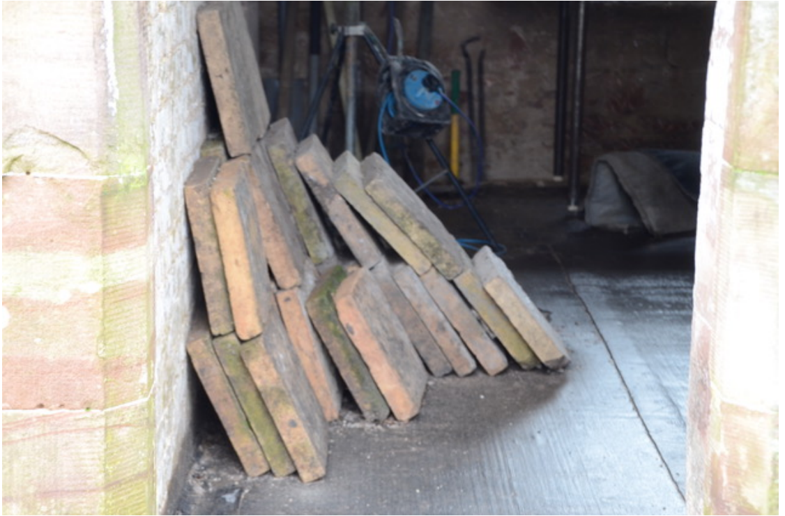
Figure 11: Stone walls and pavings under renovation.
