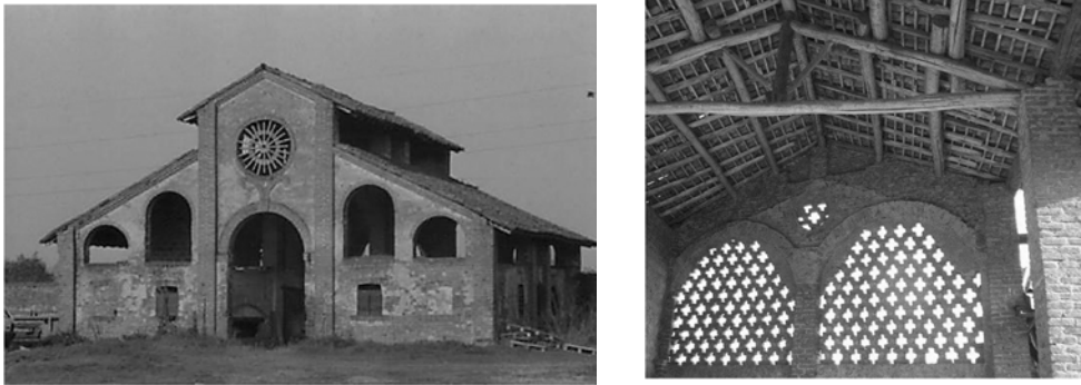
Fig. 5. On the left, the stable-barn type ( stalla-fienile ), very similar to churches with weak perforated walls ( a gelosia ), on the right.
