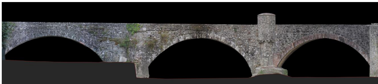
Figure 7. Orthophoto of the bridge.
