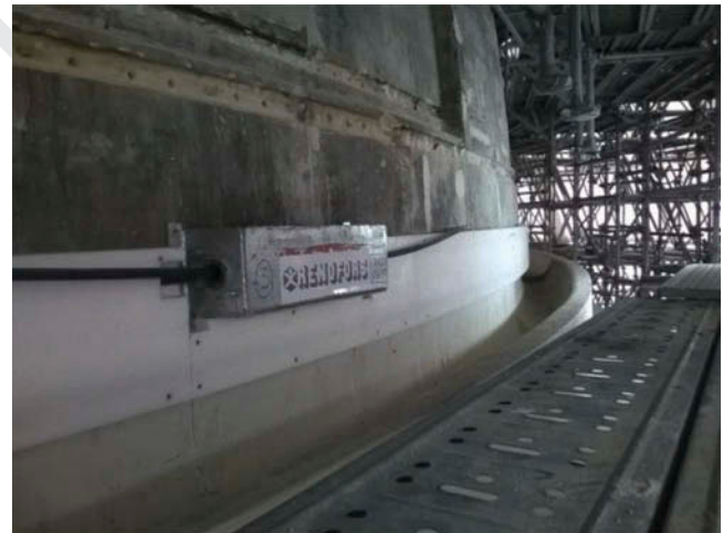
Figure 16. The new iron hoopings, realized by two pre-tensioned high resistance cables, recently added around the French Pantheon dome.
